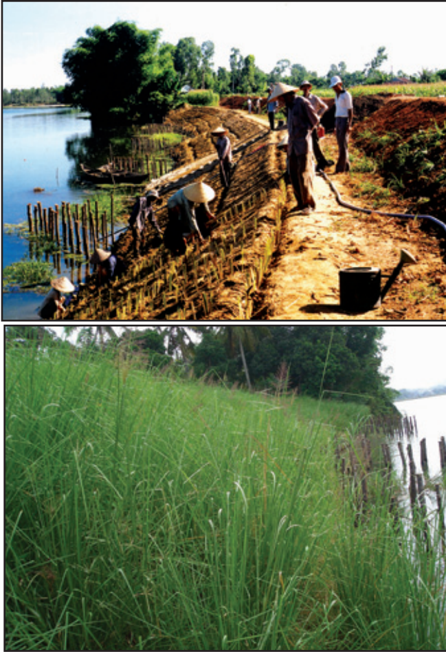
Photo 13: Upper: Community members plant vetiver; lower: November 2005: bank remains intact following the flood season.
