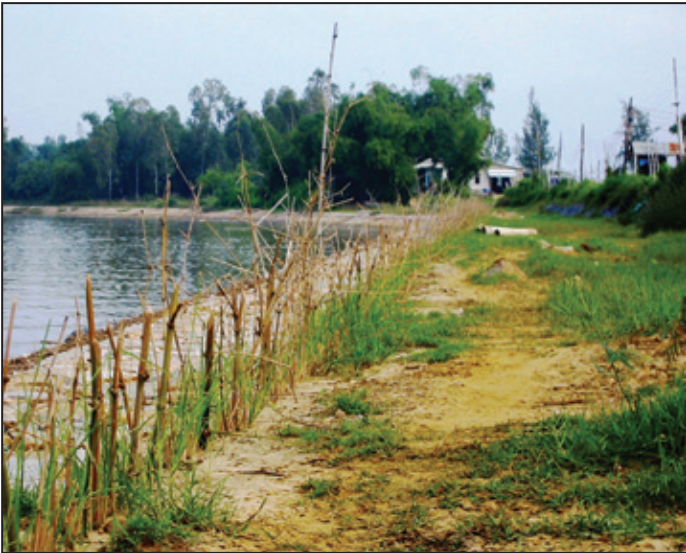
Photo 9: Upper: March 2002: VS trial at the edge of a shrimp pond, where a canal drains flood water to Vinh Dien River; lower: November 2002: mass planting combined with rock riprap to protect bank along Vinh Dien river.
