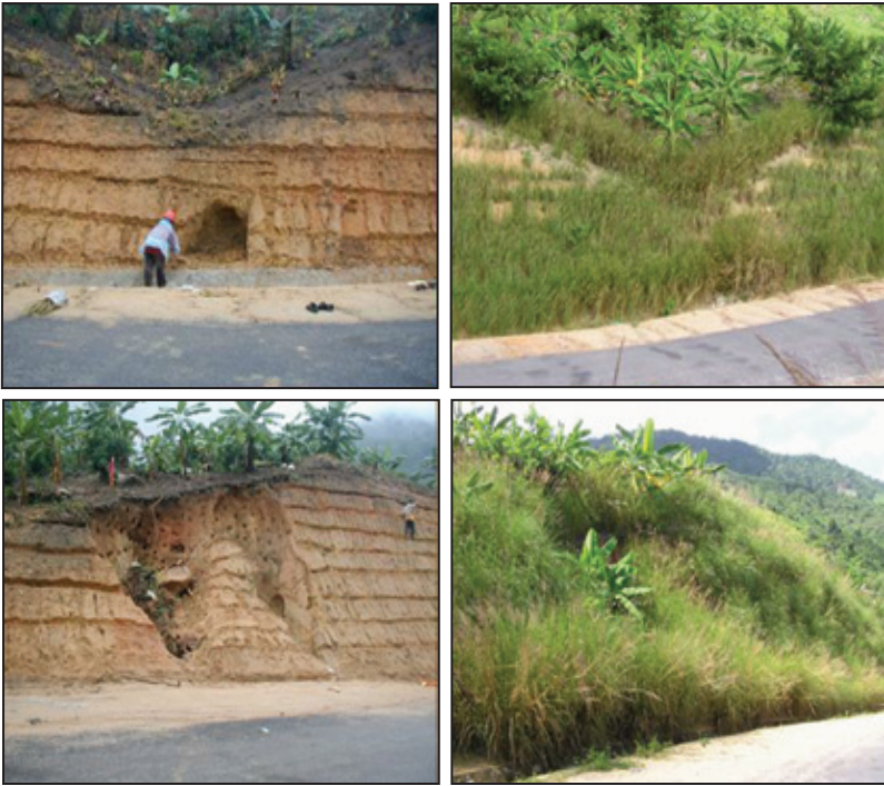
Photo 28: Pham Hong Duc Phuoc, a road protection project in Khanh Hoa province, road to Hon Ba): left two photos: severe erosion on newly built batter occurs after only a few rains; right two photos: eight months after vetiver planting: Vetiver stabilized this slope, totally stopping and preventing further erosion during the next wet season.
