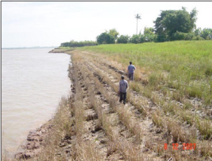
Photo 18: Flood water started coming up (upper); and dead looking vetiver on lower slope after water retreats (lower).
