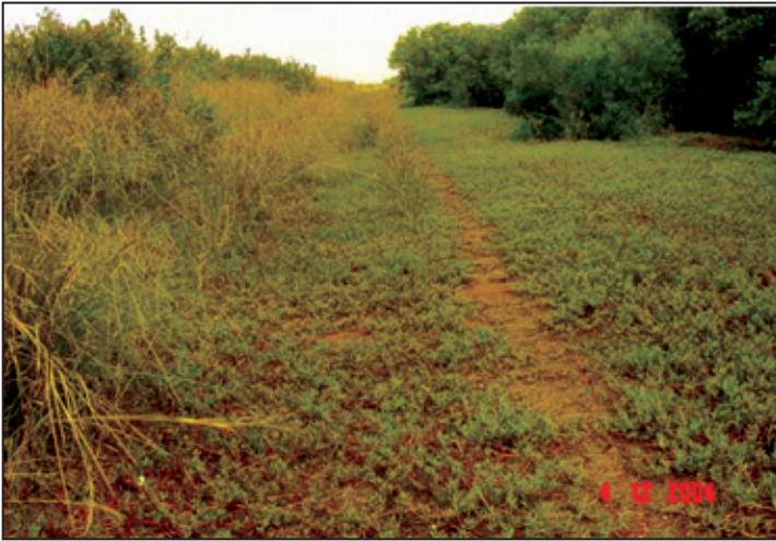
Photo 23: Planted behind natural mangrove on an acid sulfate soil sea dike in Go Cong province, vetiver reduces surface erosion and fosters the re-establishment of local grasses.
