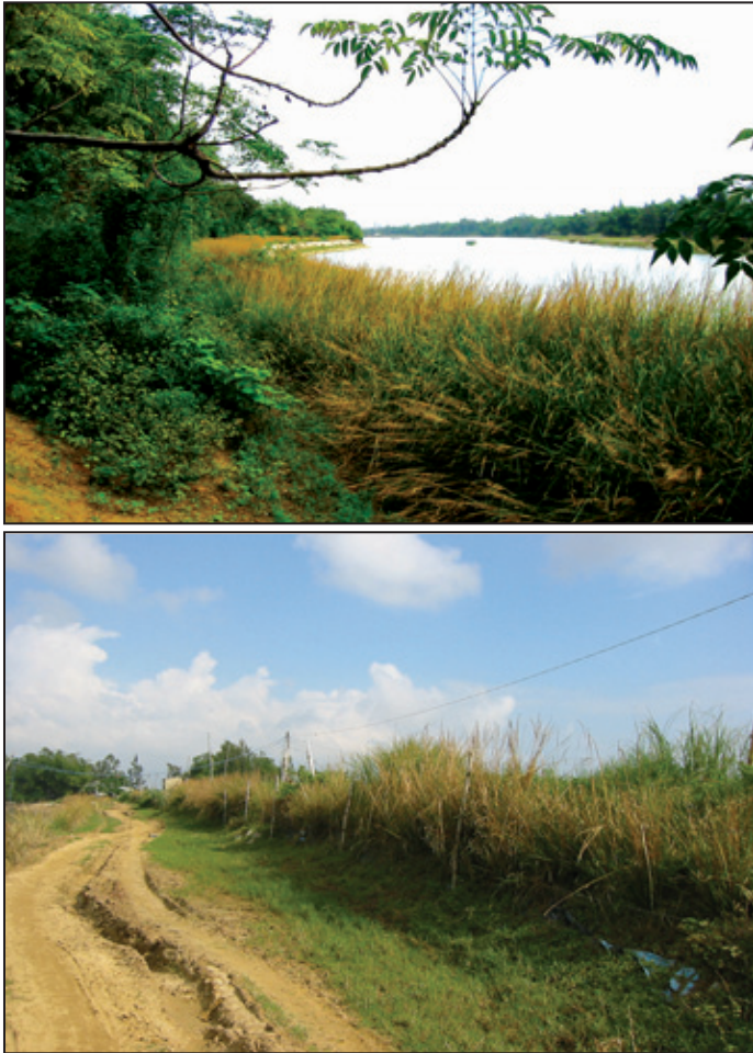
Photo 8: Upper: December 2004: Vetiver, combined with rock riprap, flourishes after two flood seasons (Da Nang); lower: planted by local farmers, vetiver protects their shrimp ponds.
