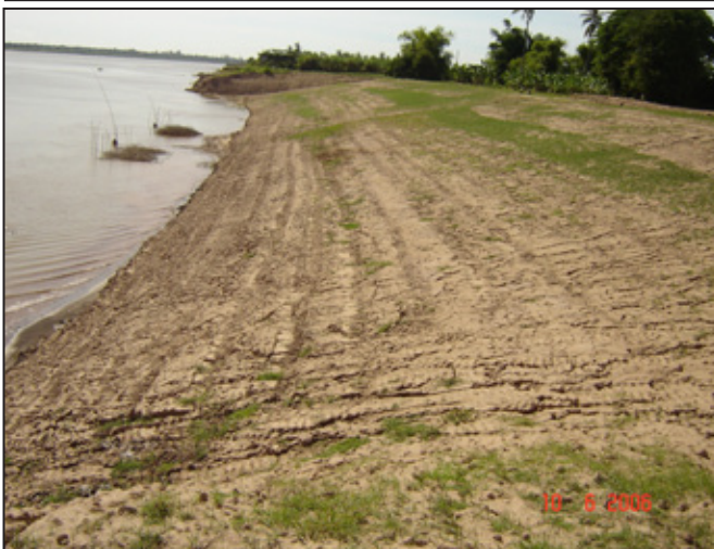
Photo 16: Eroded bank before (upper) and after earthwork (lower).
