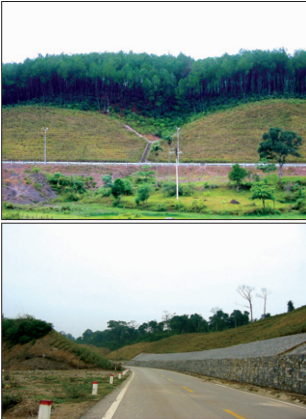
Photo 25: Upper: Vetiver stabilizes cut slopes along the Ho Chi Minh Highway; lower: both alone and in combination with traditional measures.
