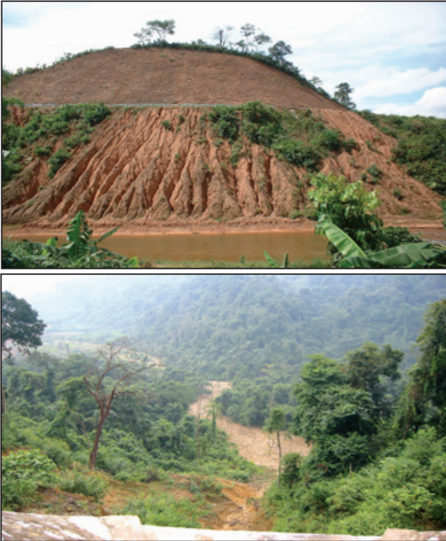
Photo 26: Upper - If not properly protected rock/soil from this waste dump will wash far downstream. Lower - impacting a downstream village in A Luoi district, Thua Tien Hue province.
