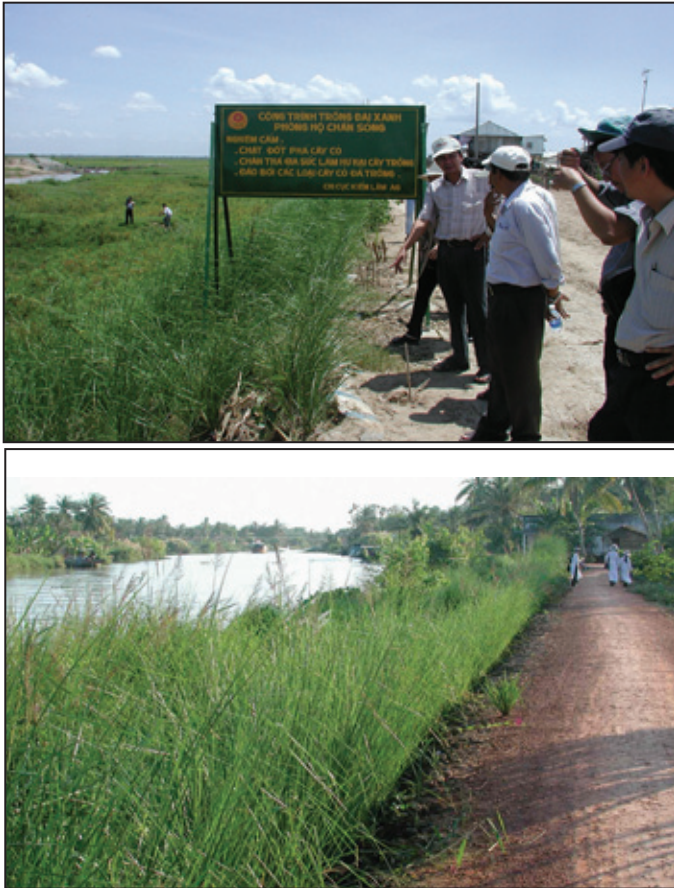
Photo 14: In An Giang vetiver stabilizes a river dike (upper), and a natural river bank (lower).
