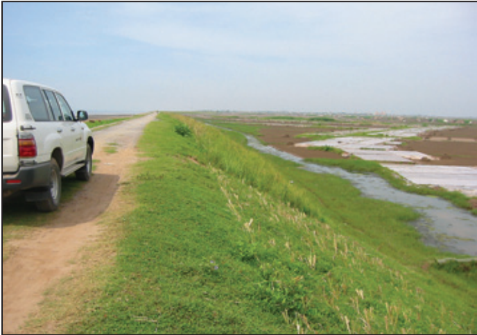
Photo 24: In North Vietnam; Upper: Vetiver planted on outer side of a newly built sea dike in Nam Dinh province; lower: on the inner side of the dike, planted by the local Dike Department.
